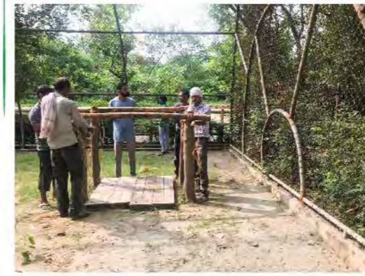
Plate 20 Resting platform in Common Leopard enclosure made with tree logs and tied with ropes
