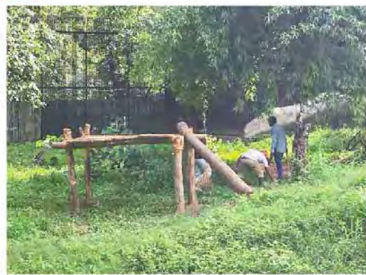
Plate 18 Resting platform in Tiger enclosure made with tree logs and tied with ropes
