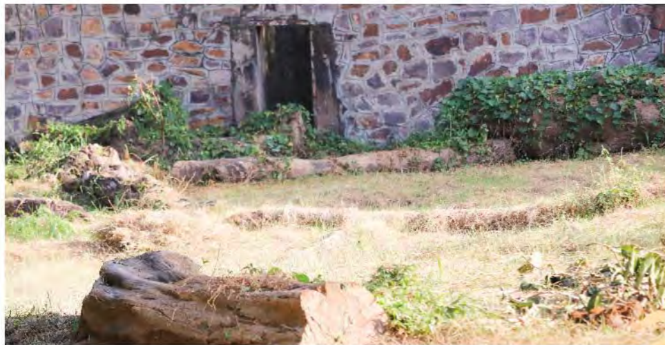
Logs Placed In enclosure
